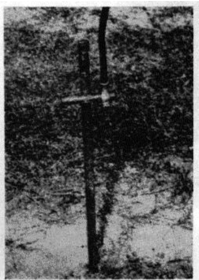
Figure 28. Installation of ground stake, semitrailer.
